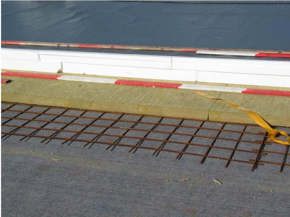
Fig. 2.15. The construction of the roof: geo-textile, iron grid, mineral wool, EPS insulation and roof foil.
