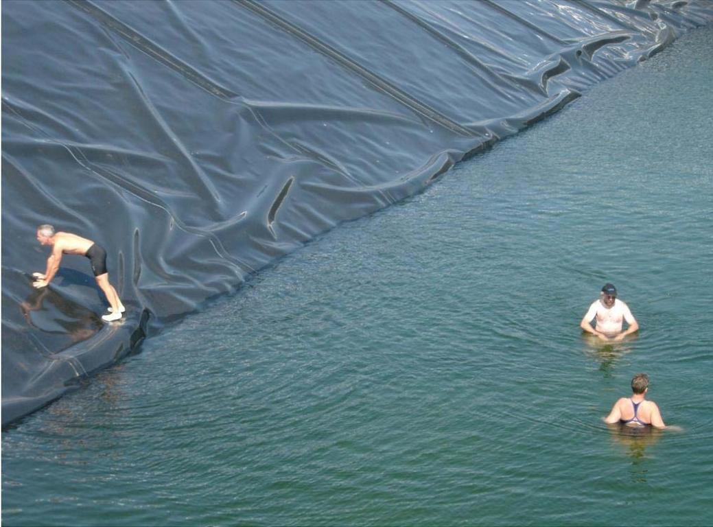
Fig. 2.12. Foldings during filling up.
